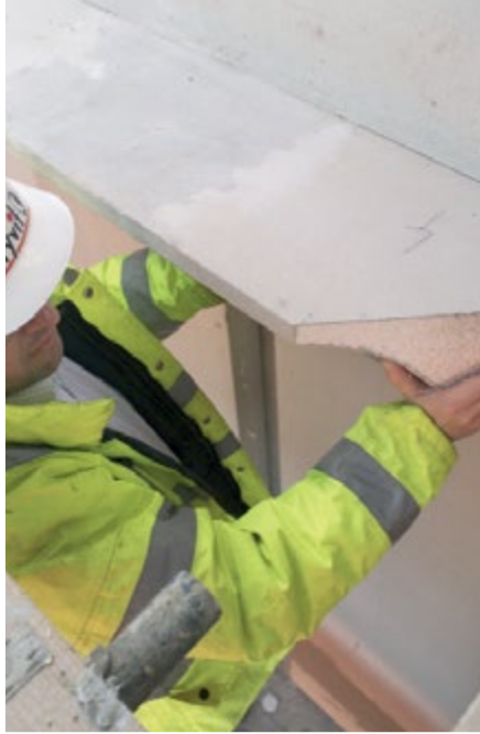
Installation of cornice
