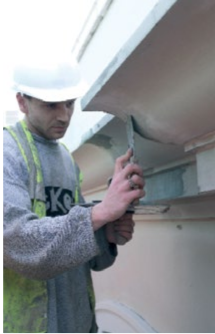
Taping of joints
