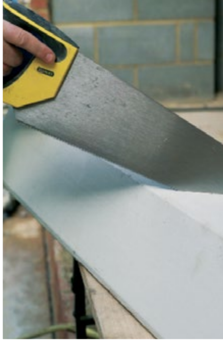
Features being cut to size on site
